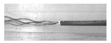
Figure 10 - Unwrap the buffer tubes.
