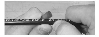
Figure 17 – Ring cut the cable jacket.
