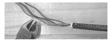
Figure 11 – Cut the central strength member to the required length.
