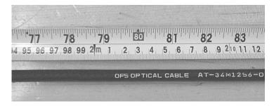
Figure 1 - Measure and mark the cable.
