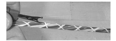
Figure 28 – Cut and remove the binder threads from the buffer tubes.
