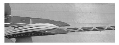
Figure 27 – Cut the dielectric strength elements to the required length.
