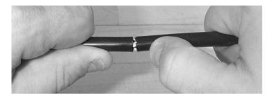
Figure 25 – Flex the cable to separate the sheath.
