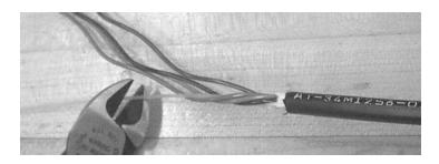
Figure 30 – Cut the central strength member.
