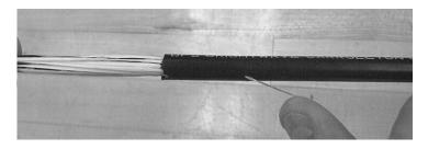
Figure 26 – Pull the ripcord to open the outer cable jacket.
