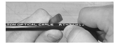
Figure 24 – Ring cut the outer cable jacket.
