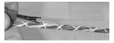
Figure 9 – Cut and remove the binder threads
