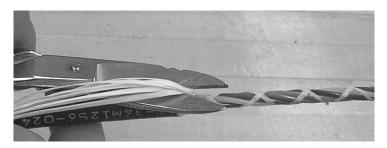
Figure 8 – Cut the dielectric strength members as required.
