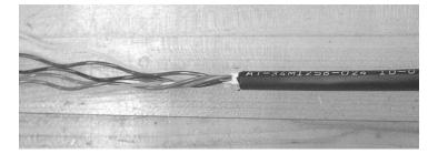
Figure 29 - Unwrap the buffer tubes.
