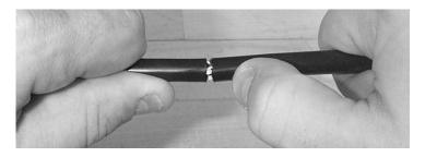
Figure 3 – Flex the cable to separate the sheath.
