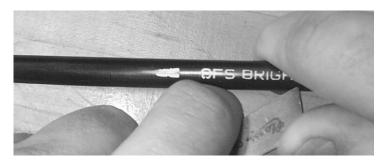
Figure 4 – If necessary, cut the cable jacket longitudinally before removal.
